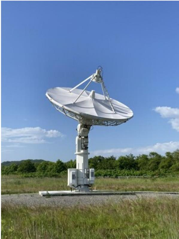
Viasat is establishing itself as a global leader in Ka-band support for low earth orbit (LEO) missions with its ability to downlink Ka-band payload data with a 7.3m full motion antenna at the Hokkaido site and is postured to support current and future government and commercial satellite programs. For Viasat, the Hokkaido ground station is a vital link in supporting high data rate remote sensing missions in polar and inclined orbits through the RTE network of Ka-band antenna systems.
